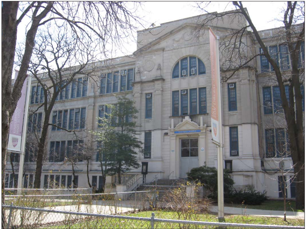
Walton High School—2780 Reservoir Avenue, north entrance 10
