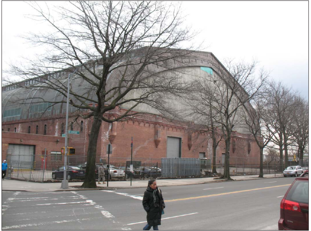
Kingsbridge Armory—View southeast on Reservoir Avenue to the Armory's west facade 5
