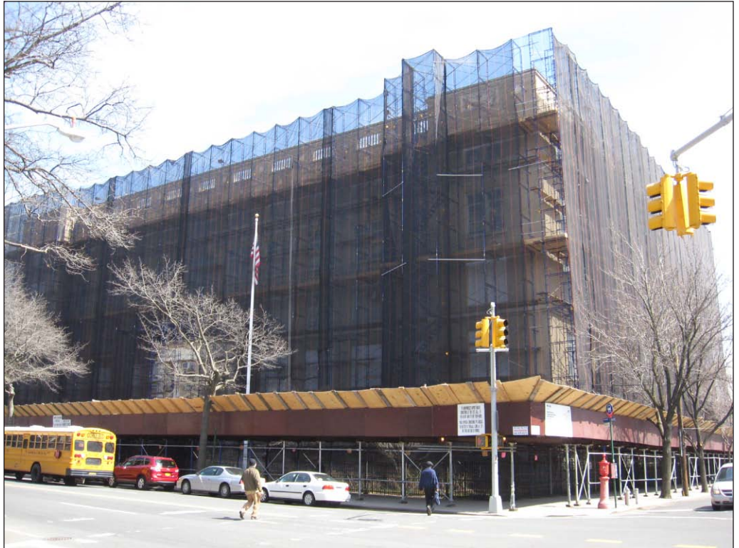
Public School 86—2756 Reservoir Avenue 11
