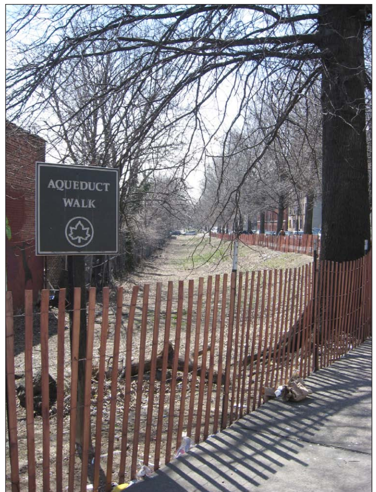
Old Croton Aqueduct— View south from West Kingsbridge Road 16
